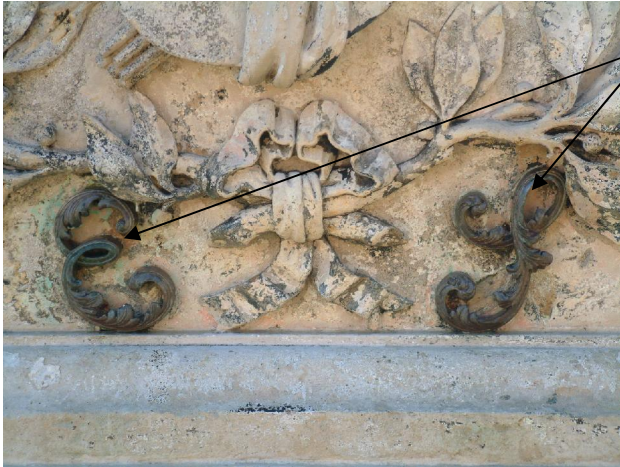
19. The bronze letters after paint removal and waxing had been carried out.
