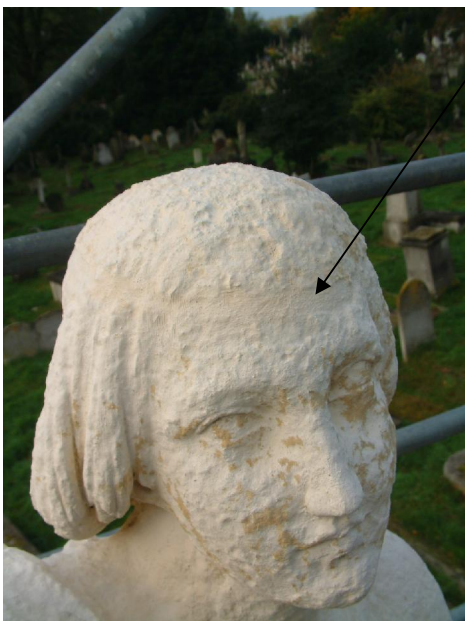
7. The finished repair to Faith's head, after two coats of lime wash (lime wash still wet).
